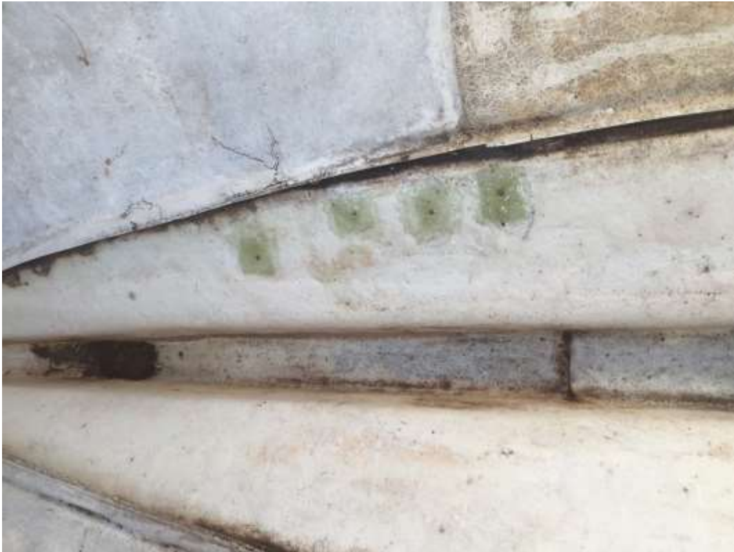
Four holes patched with fibreglass resin and matting (8 th November 2019) Two handrails completely stripped and re varnished (July 2019)
