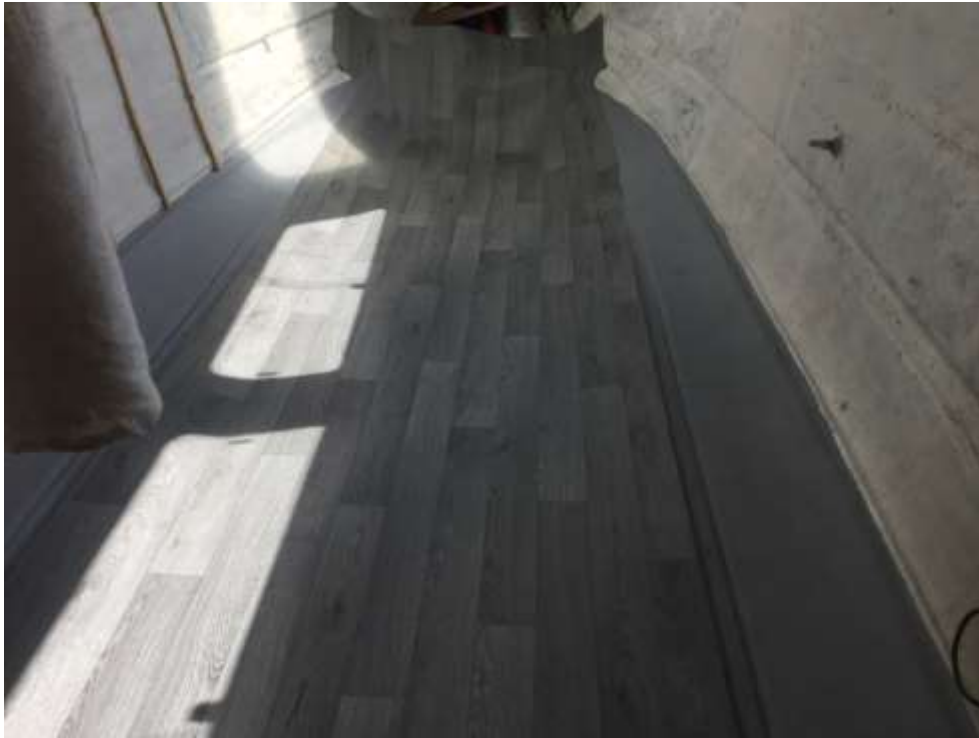
Laying the vinyl flooring (24/8/20)
