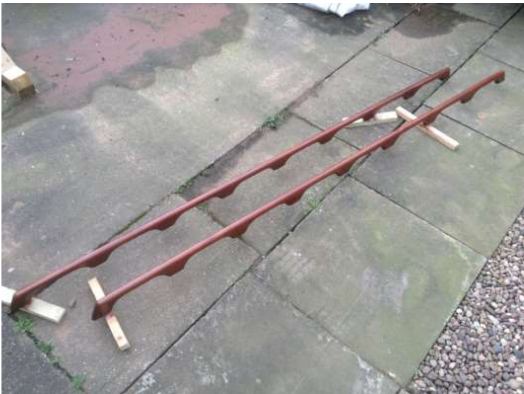
Four holes patched with fibreglass resin and matting (8 th November 2019) Two handrails completely stripped and re varnished (July 2019)
