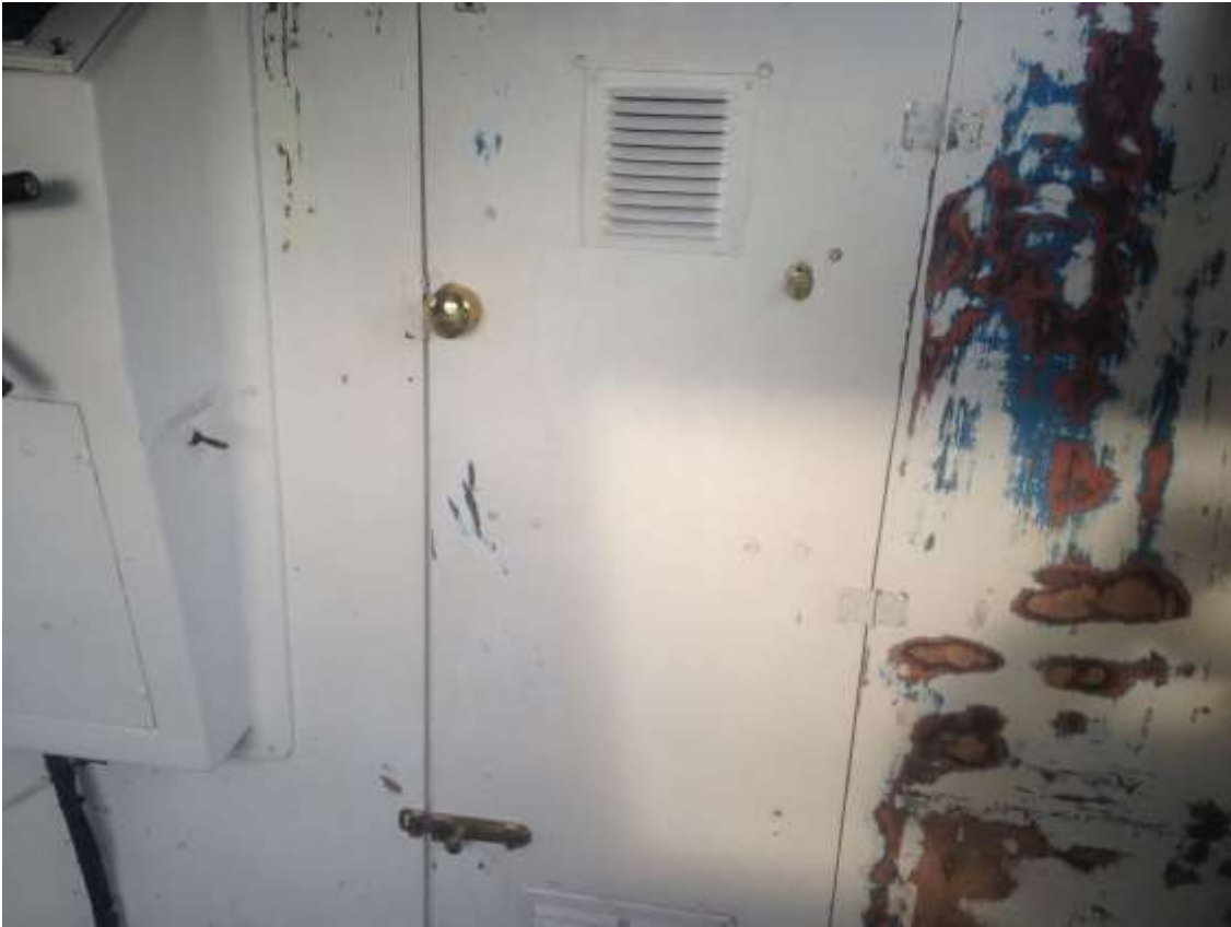
Starting to sand the cabin wall. 10/11/2017
