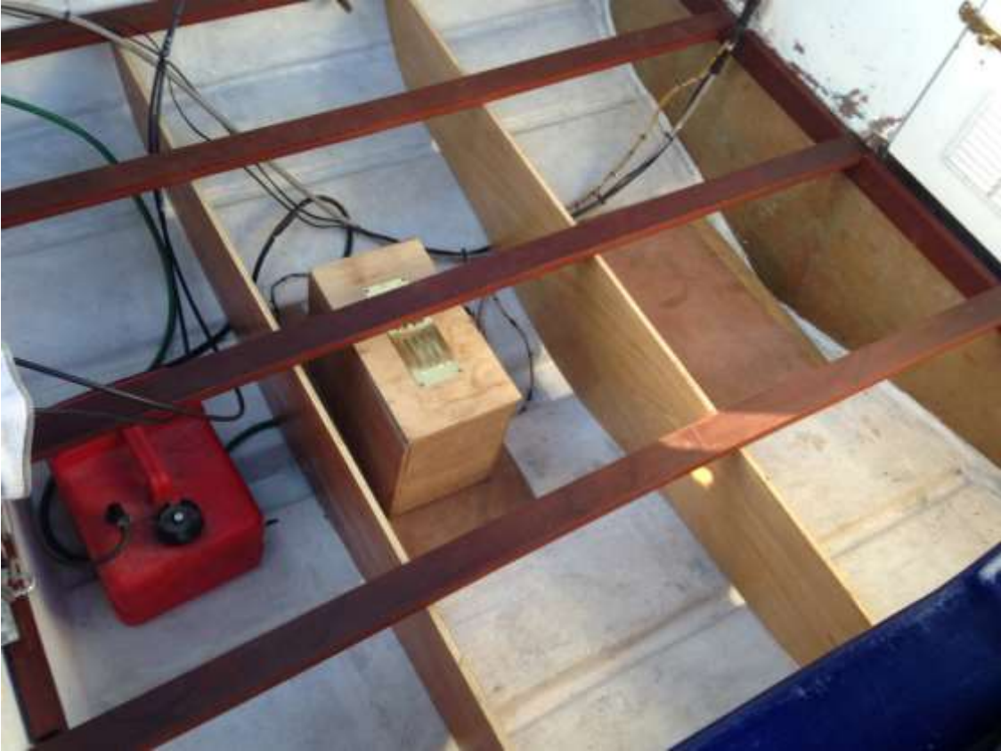
Last temporary fitting of the stringers and floor supports. 30/11/2017
