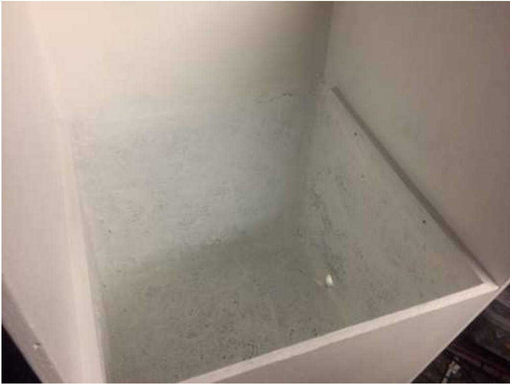
Glass fibre applied and then painted inside of gas locker 22/3/2018
