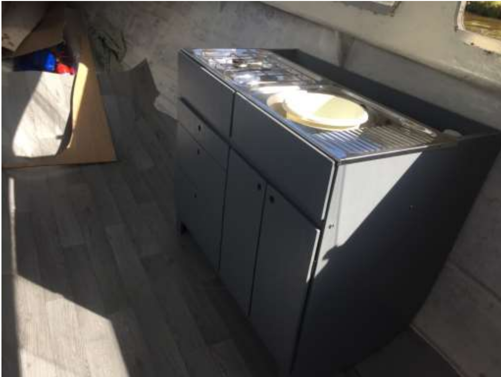
Installed Kitchen unit (24/08/20)
