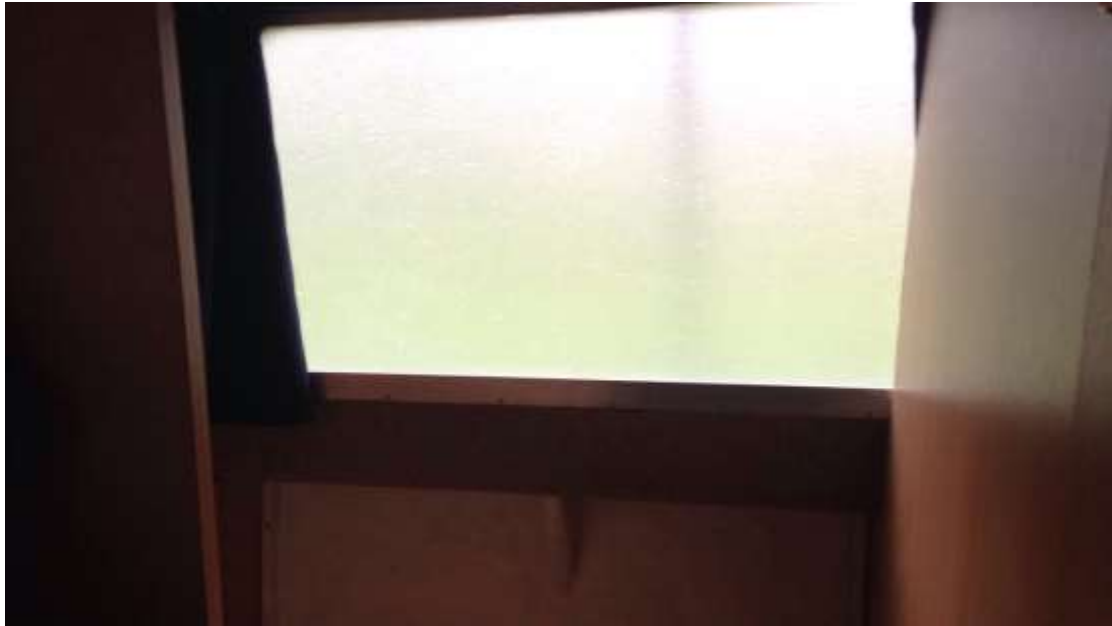
Obscure window film fitted to toilet window.
