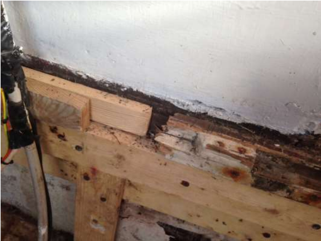
Patched up wood frames and when trying to remove to act as template all the plywood had rotted between the fiberglass. 27/10/2017
