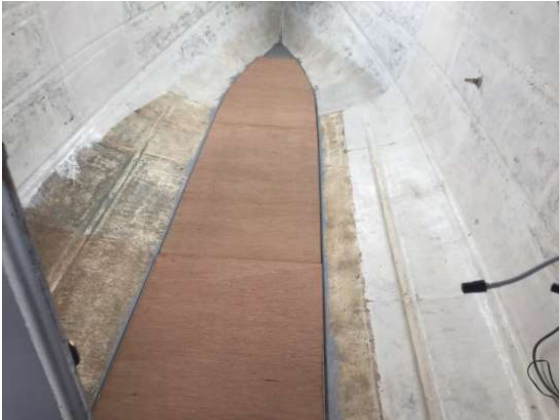
18mm plywood floor primed underneath & bonded to fibreglass (2/7/2020) Whole floor area painted with grey primer (2/7/2020)
