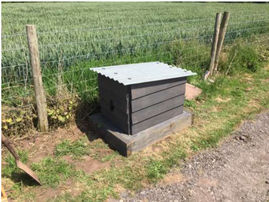
Generator box installed (07/06/2018)
