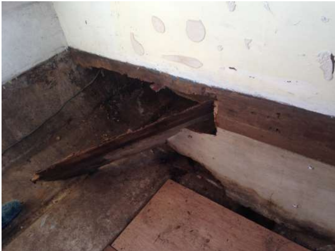
Even the rear bulkhead fell apart when removing.
