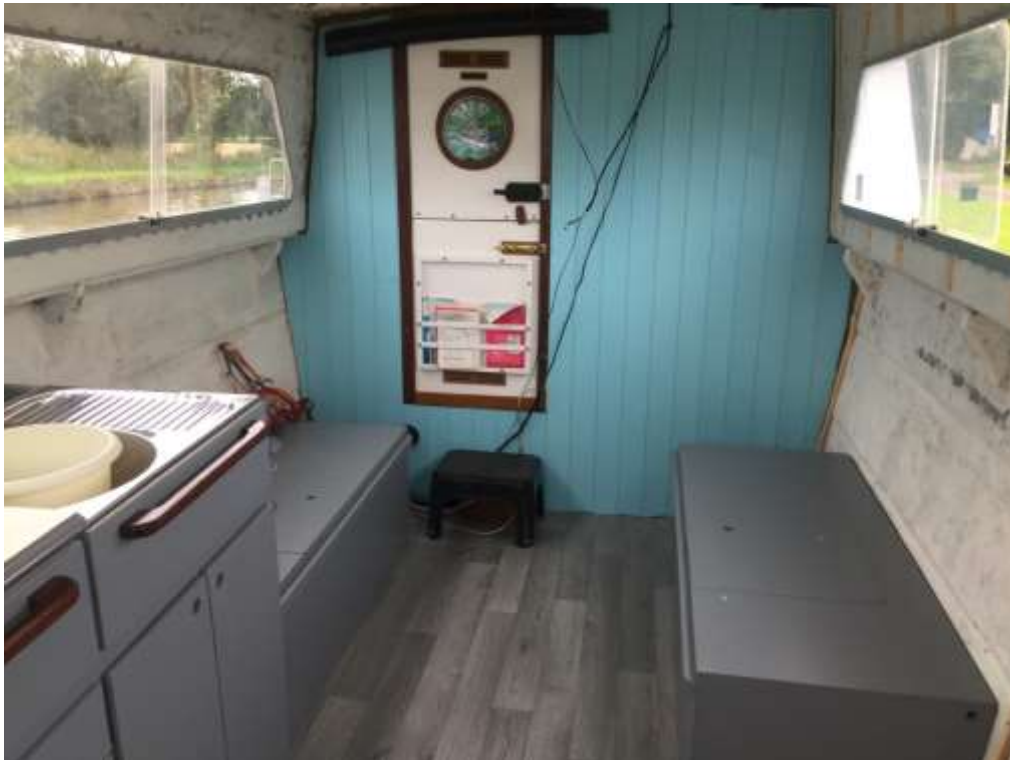
Sofa beds installed and cabin wall clad (04/09/20)
