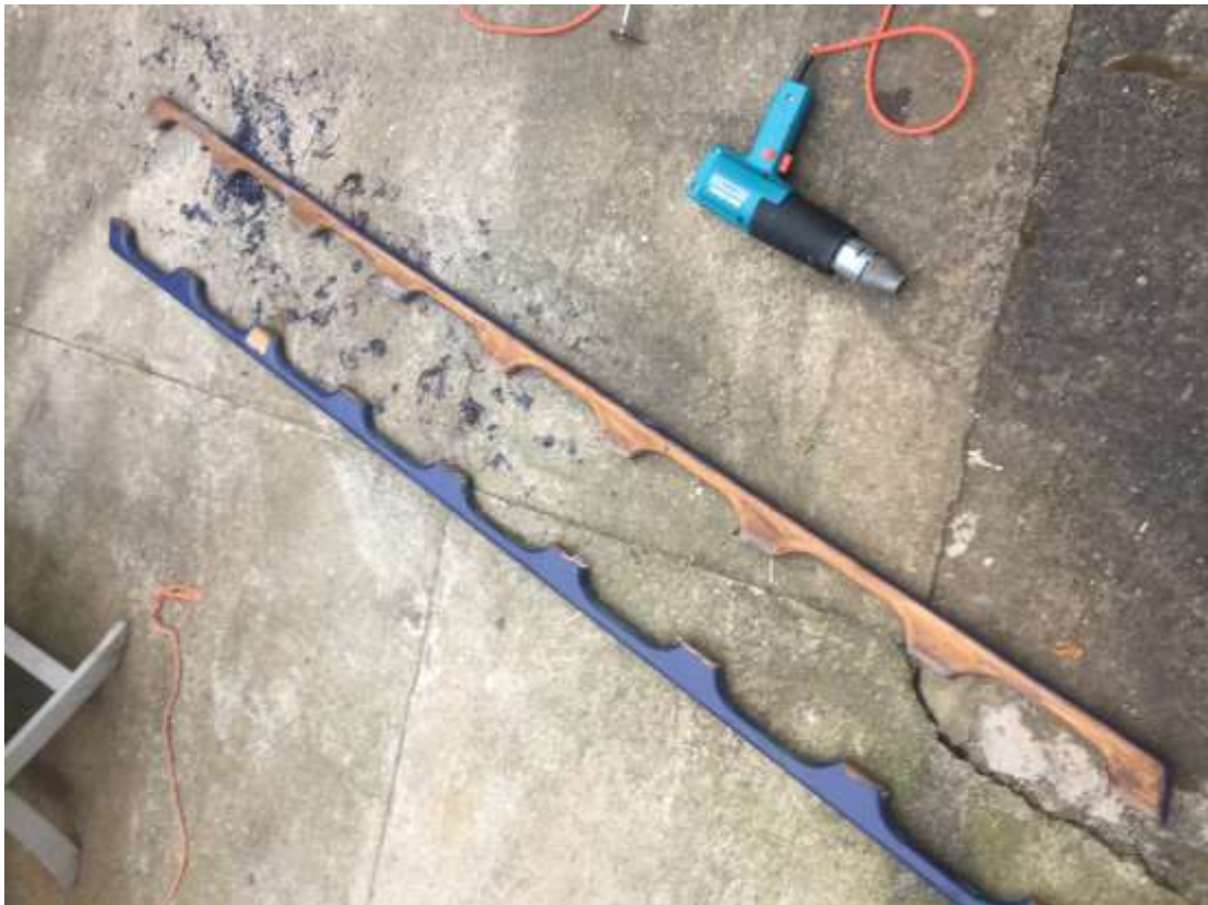
Continued sanding Striping paint off the hard wood hand rails (July 2019)
