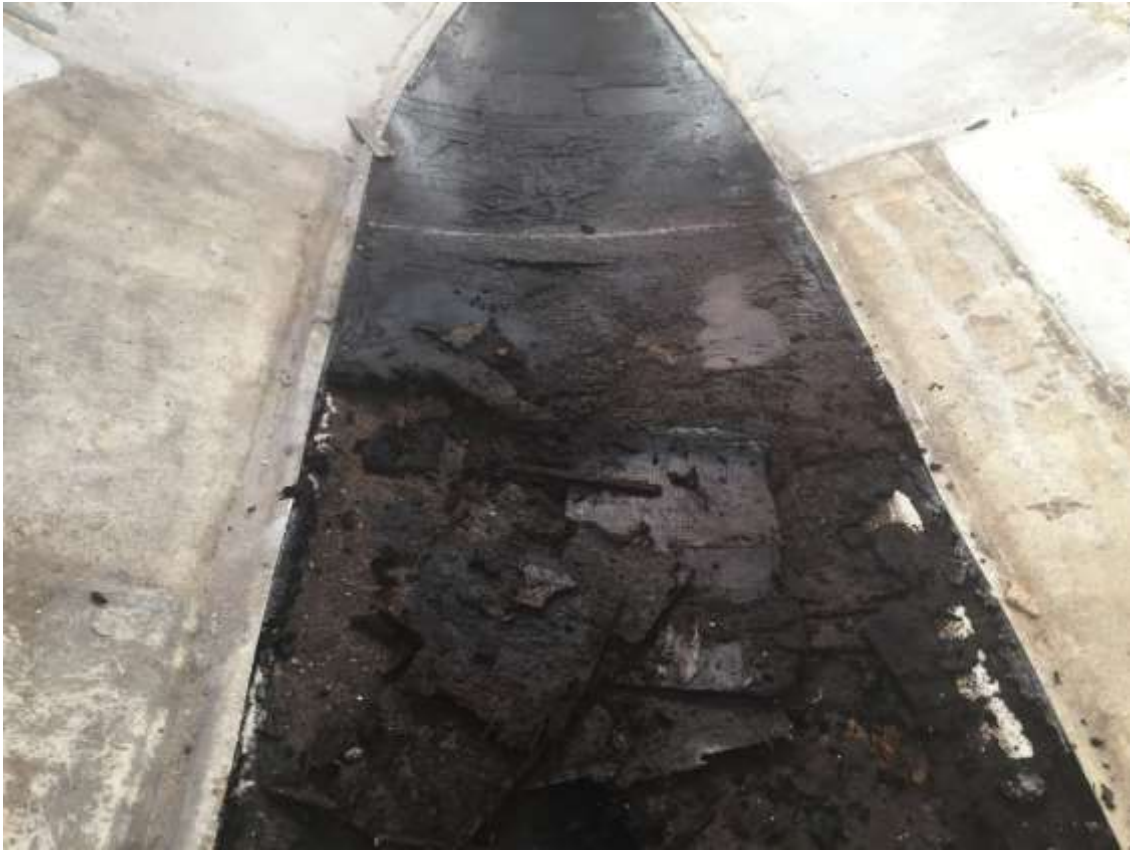
Originally there had been plywood between fibreglass and sand but this had rotted completely.
