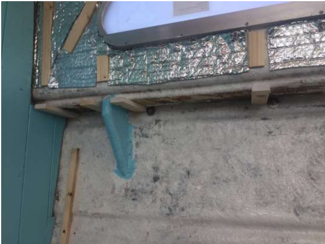
Front battened & insulated and cladding started (05/09/20) Hull side walls and knee insulated and battened (09-11/09/20)
