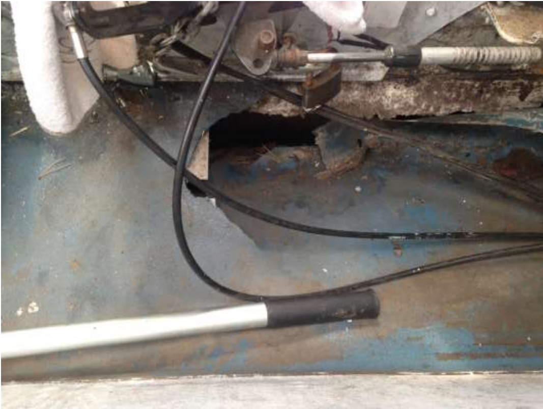
Plywood floor in storage area was hiding two previous rotten floors and their vinyl covering.
